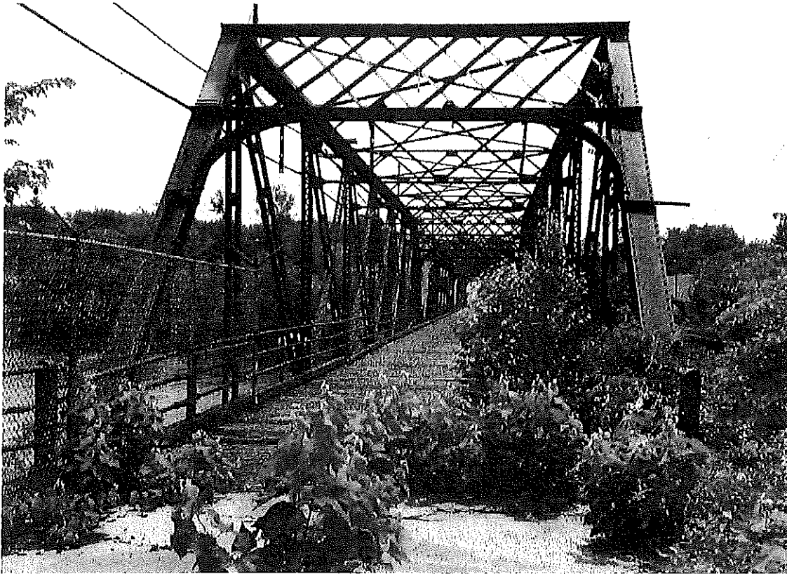
Lilac Bridge over the Merrimack River Veterans Drive Hooksett, NH Br. No. 083/150, NHDOT Project No. 29655 Bid Item No. 1, 2, and 3
